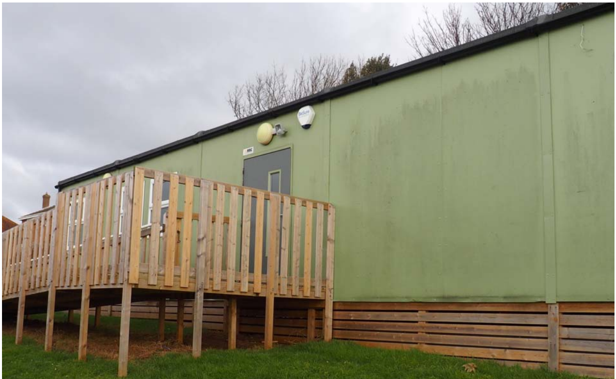
Photograph No. 08 - Portacabin building which offer 'negligible' bat roost potential.
