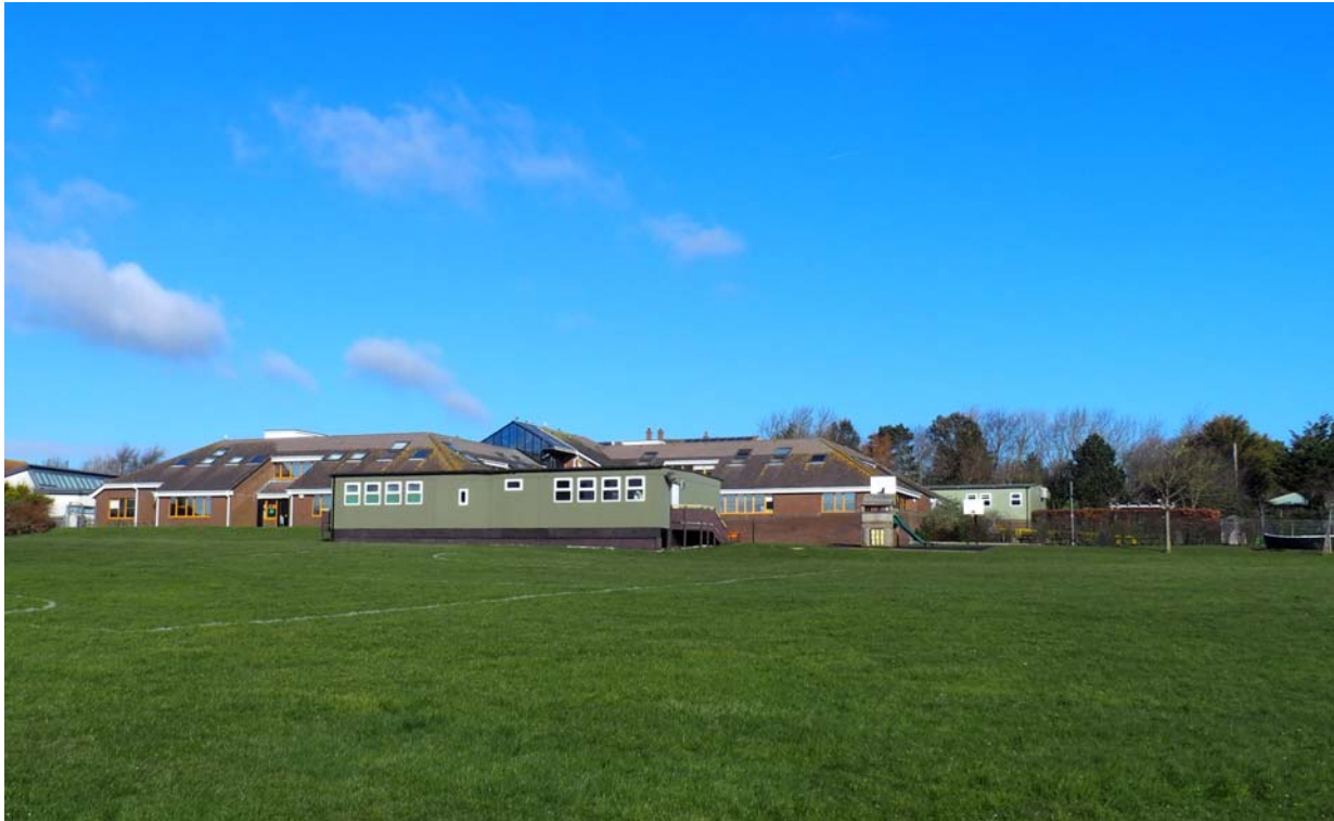
Photograph No. 01 - View across the site looking towards the main school buildings.
