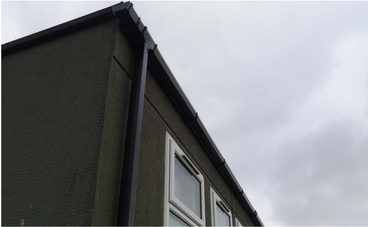
Photograph No. 09 - Portacabin building which offer 'negligible' bat roost potential.
